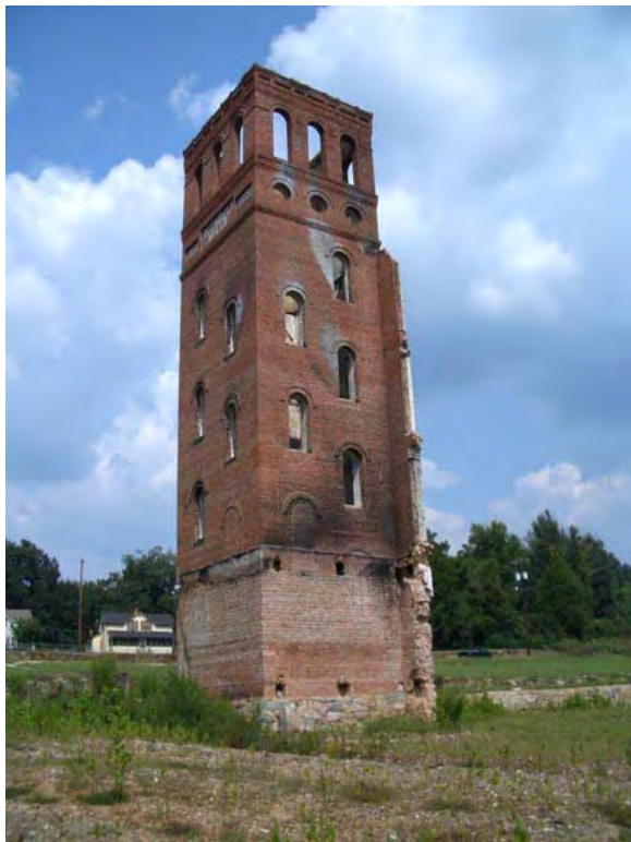
One of the two remaining towers at the site of the Glendale Mill
